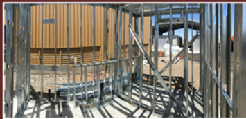
$998K Newberry Springs Station Structural Framing-In Progress
