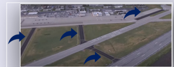
Joint Base Taxiways A, C & D
