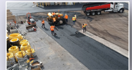
Asphalt & Concrete Paving
